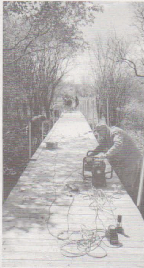
Construction of the Boardwalk
